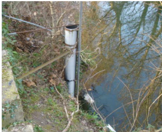
Figure 9 : photo emplacement station mobile pont A8
